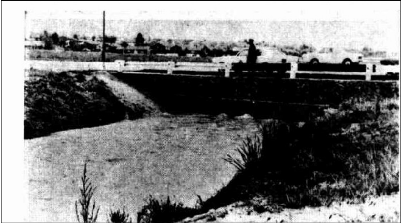
Water rushes into the pipes under the culvert at the Melrose Drive, Yamba Drive intersection in the Woden Valley yesterday after soaking rain all day yesterday.
