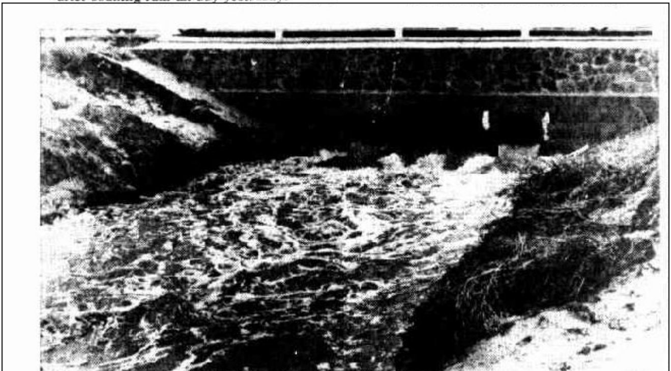
In this picture, taken at the same time, the outlet on the other side of the culvert discharges the water into the storm water channel at a lower level.
